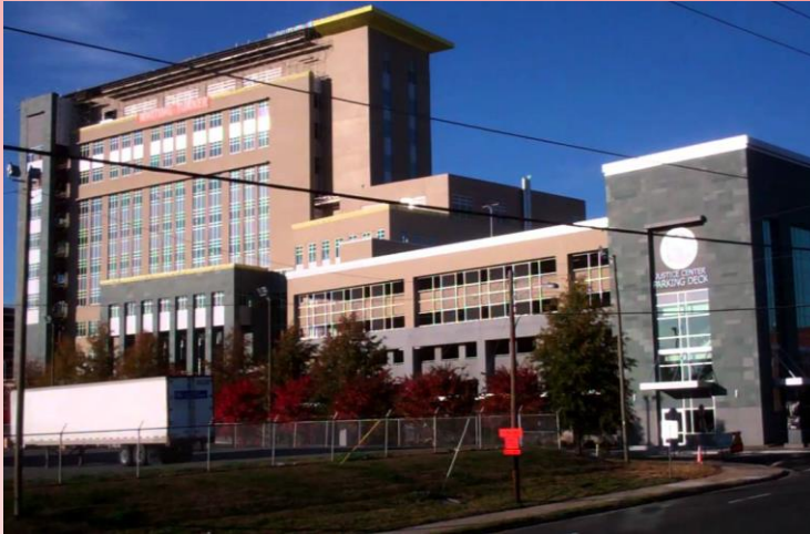
Durham County Judicial Center Parking Deck
